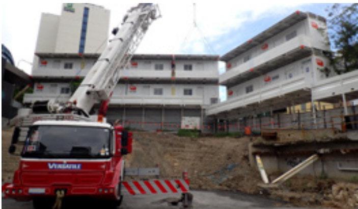
Loading overhead protection at the start of the project
