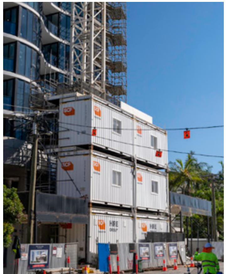
The project further into the build, with the structure taking shape
