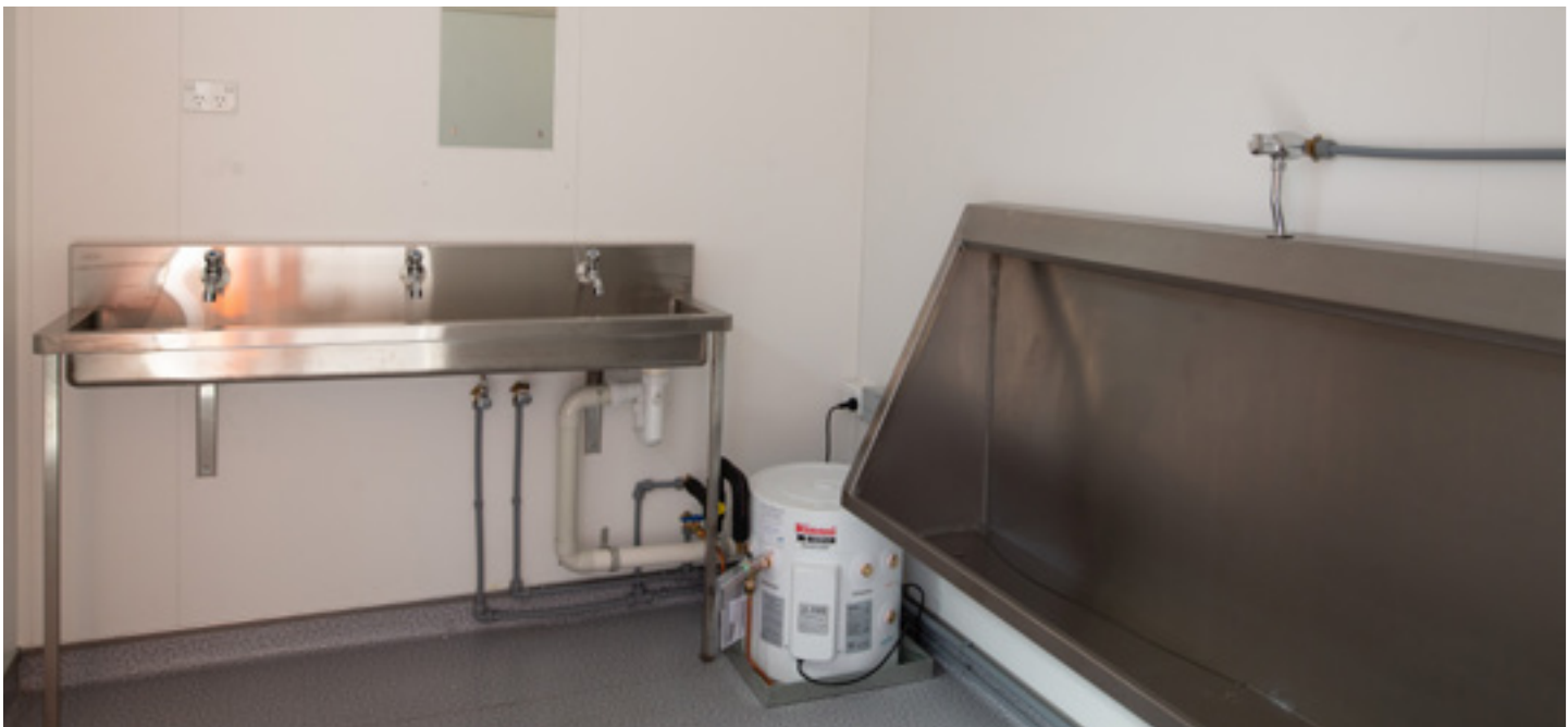
Below: The main block has ample wash space, so your team can get it done quickly. It also includes hot water for those cold days.
