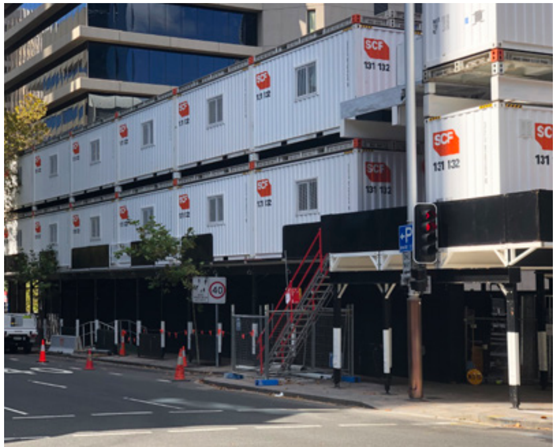
This site includes ablution blocks, site offices, lunch rooms, first aid rooms, a shower block and change rooms.
