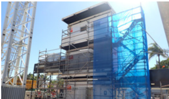
Various Site Sheds deployed to ensure the project runs smoothly
