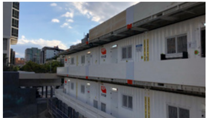
Site constraints meant a double stack with 40ft containers was required
