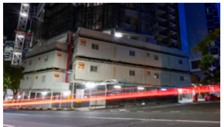
SCF Site Sheds visible at night
